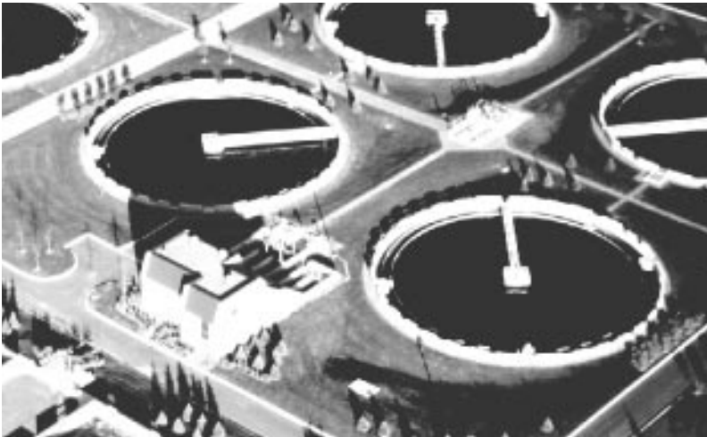
Figure 8. Water treatment facility
